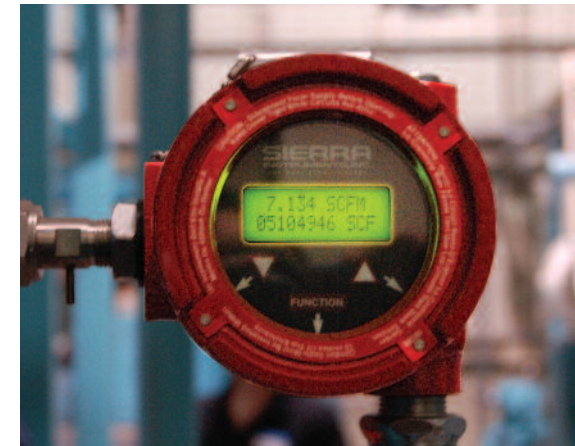
Sierra Steel-Mass™ 640S on a digester tank
